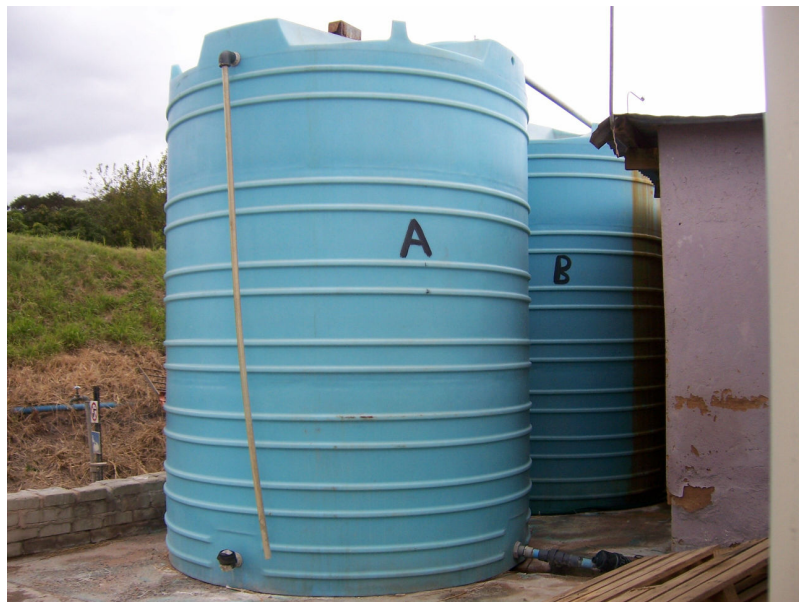
Simple A and B tank configuration. Fertilizer materials must be separated to avoid chemical interactions in the tanks.
