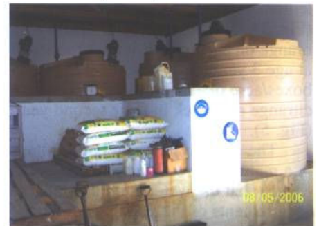
Fig. 1. Inside an Open Hydroponic System control facility in South Africa showing the piping, controller, pumps (above) and the fertilizer tanks (below).
